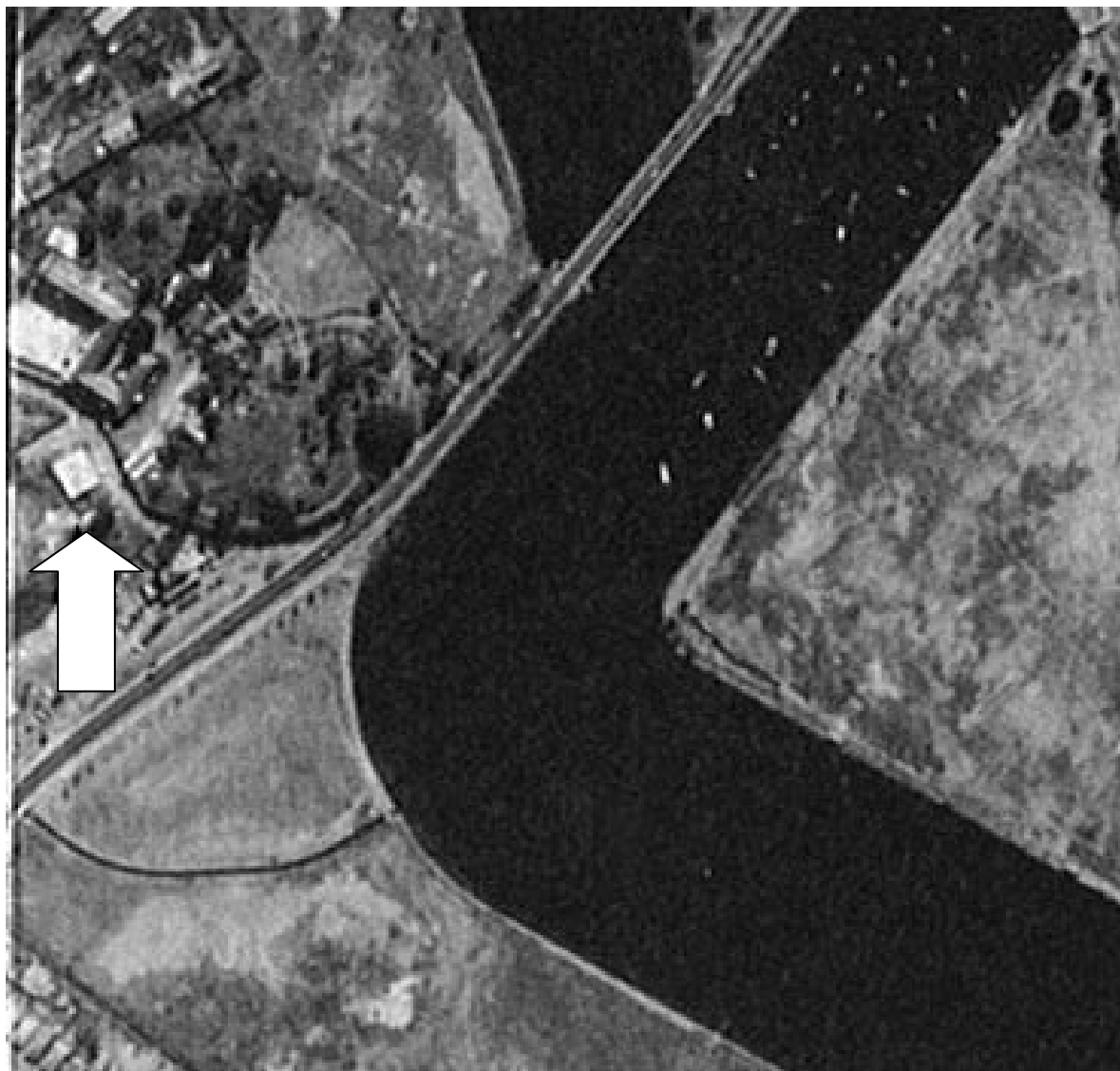
Figure 3.7 1951 photograph with the first of the buildings currently on site, on the corner of Arncliffe Road, arrowed. From this period the site was gradually developed as an industrial area. Note also that the Highway has been realigned in comparison to Figure 3.5 and 3.6. (Source: Department of Lands)
