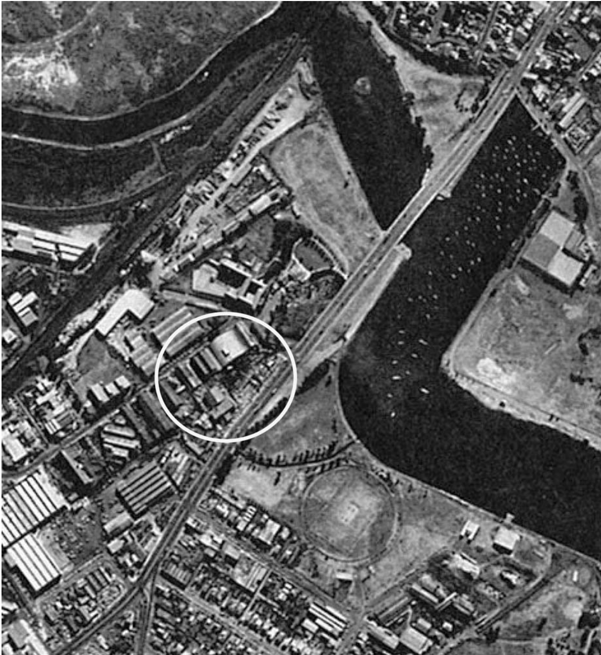
Figure 3.8 1970 aerial photograph with the study area circled. Note in comparison to Figure 3.7 the site is now fully developed with light industrial sheds and warehouses. (Source: Department of Lands)
