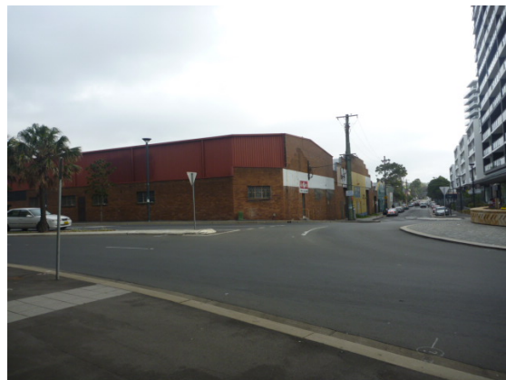
Figure 10 The existing masonry façade of this structure, 96 Arncliffe Street, is proposed to be retained and modified with new openings to allow truck access to the proposed delivery dock. (Source: GML 2009)
