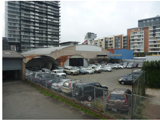
Figure 8 Rear view of warehouses facing Arncliffe Street. Wide span and curved roof of 90–92 Arncliffe Street shown. (Source: GML 2009)
