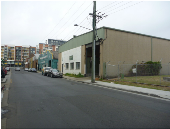
Figure 5 The westernmost structure on the Arncliffe Street side of the site. This structure is proposed for demolition and replacement by a new entry and exit road. (Source: GML 2009)
