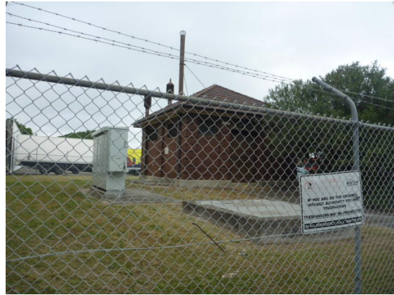
Figure 6 Sydney Water pumping station adjacent to the subject site on the western elevation at Arncliffe Street. (Source: GML 2009)
