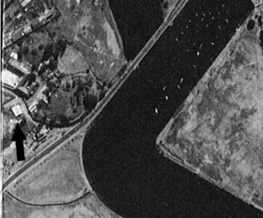
Figure 7 1951 photograph with the first of the buildings currently on site on the corner of Arncliffe Road (arrowed). From this period the site was gradually developed as an industrial area. Note also that the highway has been realigned (compare to Figures 3.5 and 3.6). (Source: Department of Lands)
