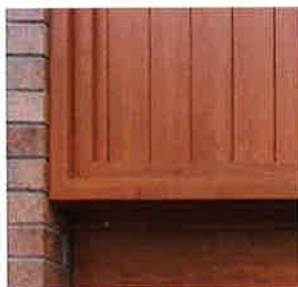
Modern, flush-closing blade profile
