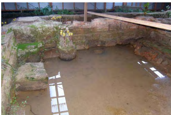
2008 flooding of the site caused some damage to the archaeology, especially the collapse of the sides of excavation trenches and the partial undermining of the foundation material below remnant brick walls
