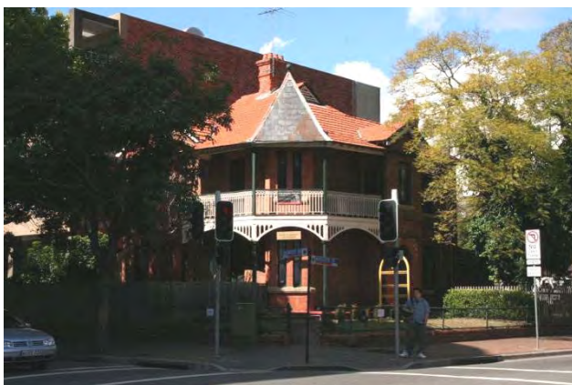
The nearest heritage listed property to the subject site is located at 41 Hunter Street, on the south east corner of Marsden and Hunter Streets, diagonally opposite the subject site.
