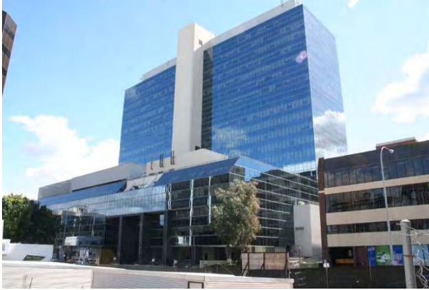
Looking north west from the subject site towards the high rise Government office building in the distance
