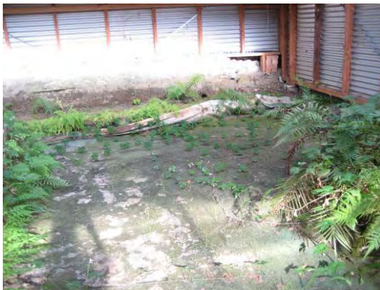
Also noted along the north side of the overall site (outside of the sheds) along Macquarie Street.
