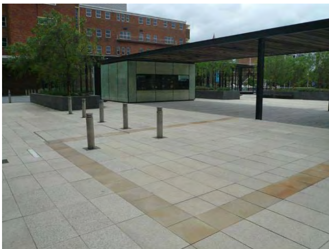
A similar paving has been used to mark the outline of another of the former hospital buildings.
