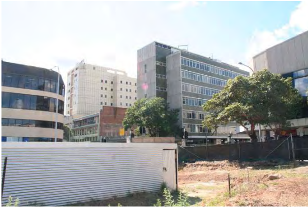
View looking south east at the medium scale commercial buildings to the south of the subject site
