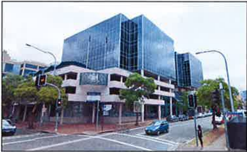
Figure 14: Corner of Hunter and Marsden Street
