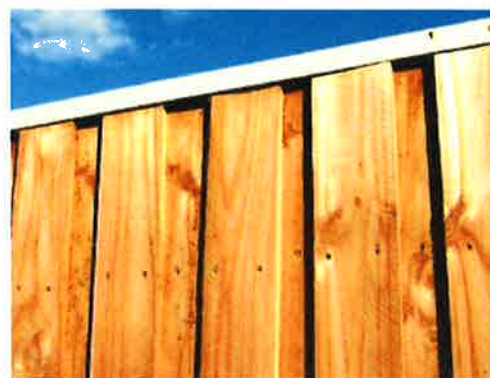
TIMBER PALING FENCE
