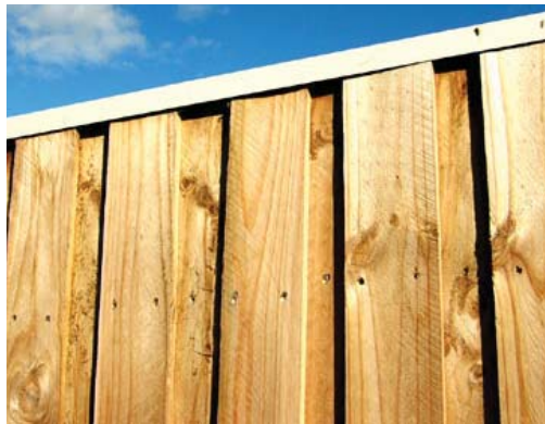
TIMBER PALING FENCE
