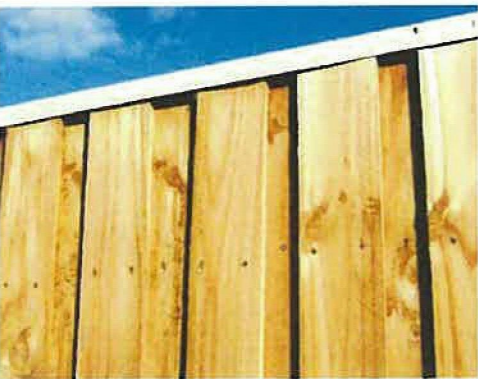
TIMBER PALING FENCE
