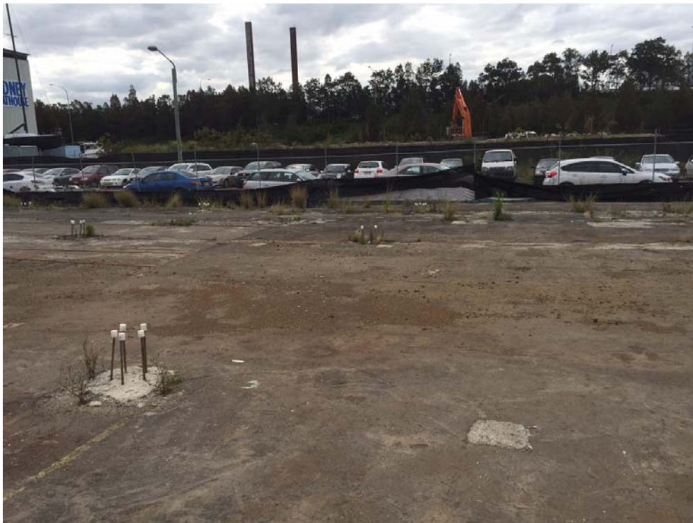
Figure 5 Completed piling works for the western building
