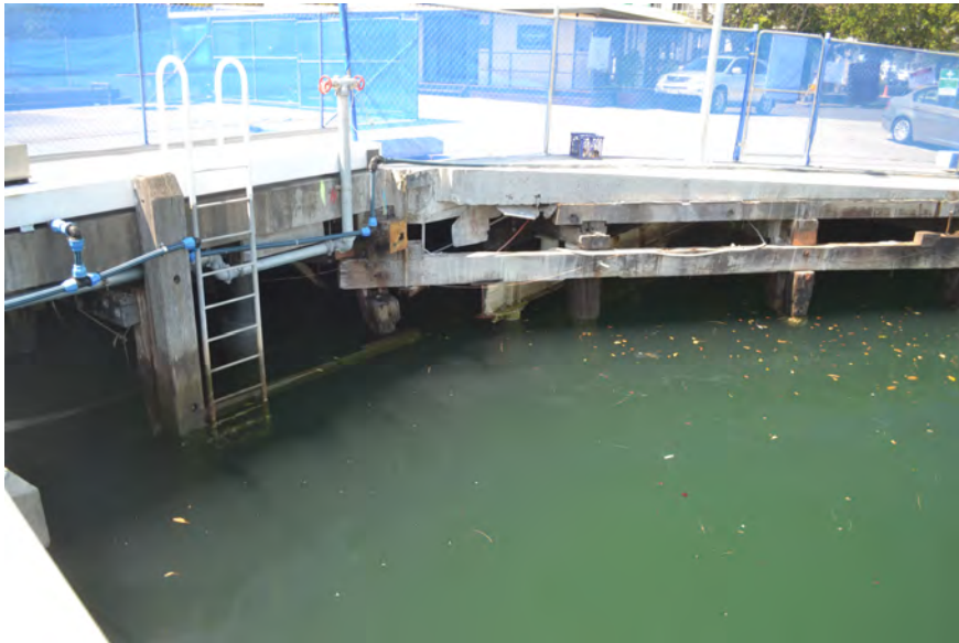
Figure 7 View of inshore marina concrete pad.
