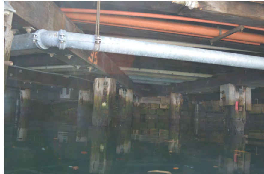
Figure 8. View under concrete pad showing sandstone rock wall inshore
