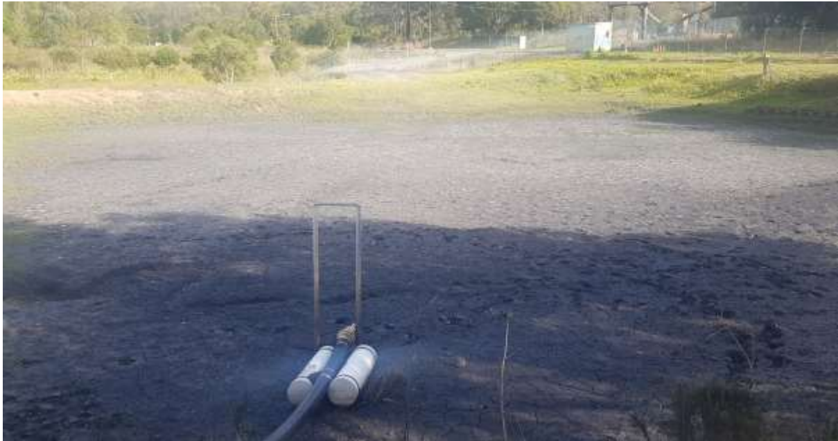
Photo 1: Settling pond with significant volume of sediment present
