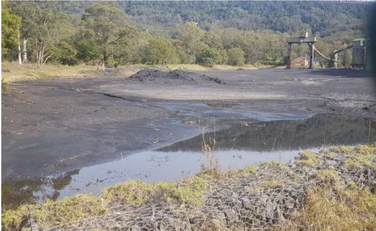
Photo 3: Settling pond with significant volume of sediment present
