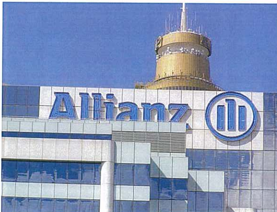
Figure 4 - View of the Allianz sign and logo at east of Darling Harbour.
