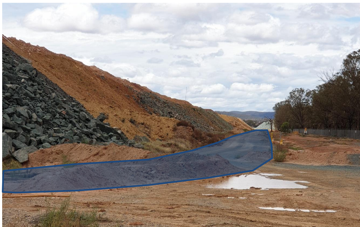
Plate 1 View of indicative additional disturbance area (blue) from southwest corner of the Residue Storage Facility looking east (Ref: Client Supplied 10 February 2020)
