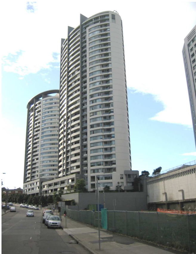
Figure 3 – Photo of the site in the fore ground with existing residential development (Epica and Altura) to the north
