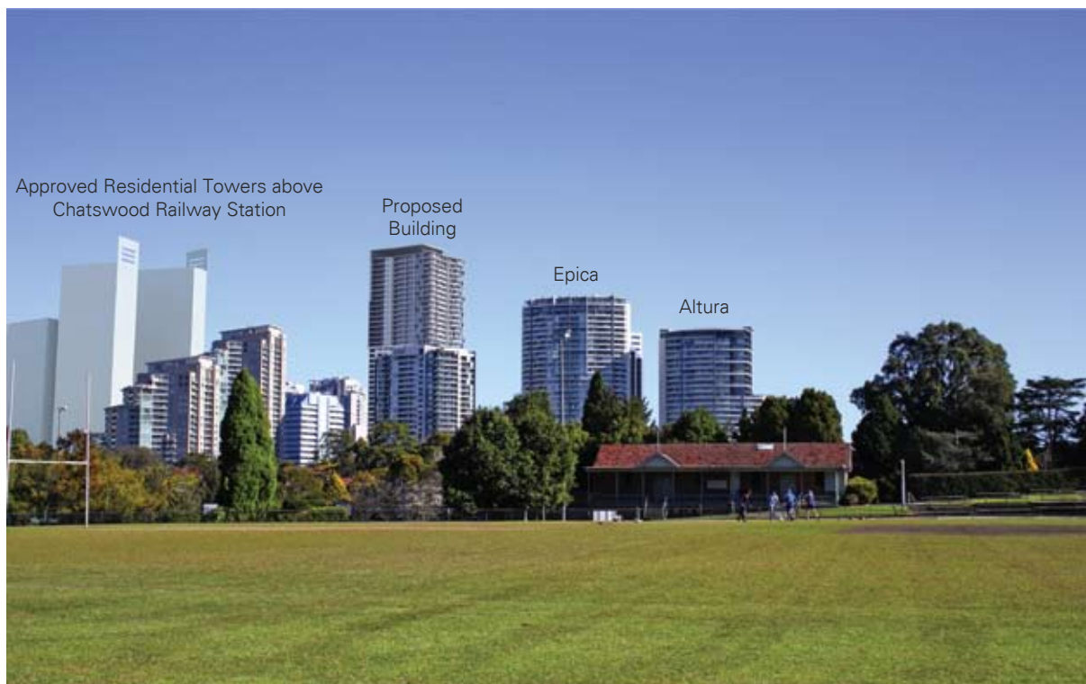
Figure 24 – Chatswood CBD Skyline as viewed from Beauchamp Park Source: Mirvac Design Pty Limited
