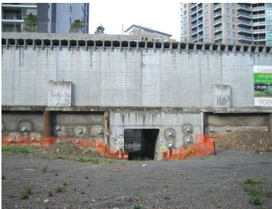
Figure 10 – Existing through site link under the RES
