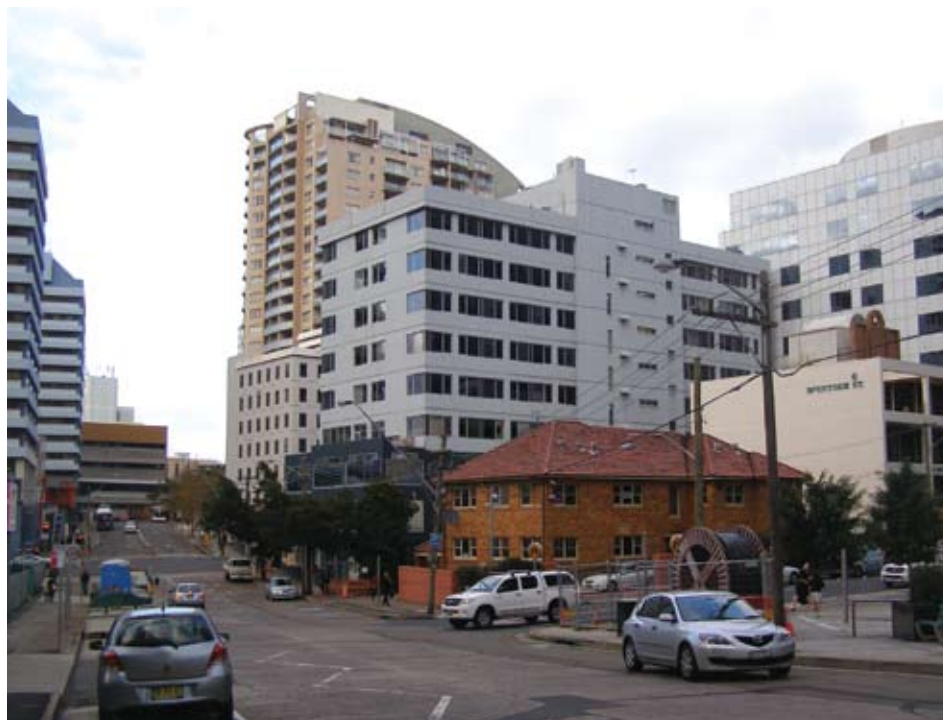
Figure 19 – Commercial buildings to the west of the site as viewed looking towards the south-west
