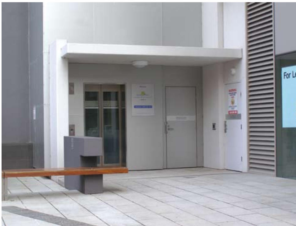
Figure 9 – Lift providing public access to the RES
