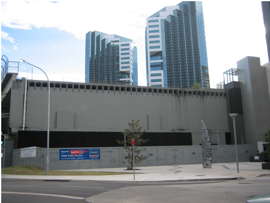
Figure 4 – Part of the site on the eastern side of the railway (surrounded in hoardings) looking west with the Zenith Towers in the background
