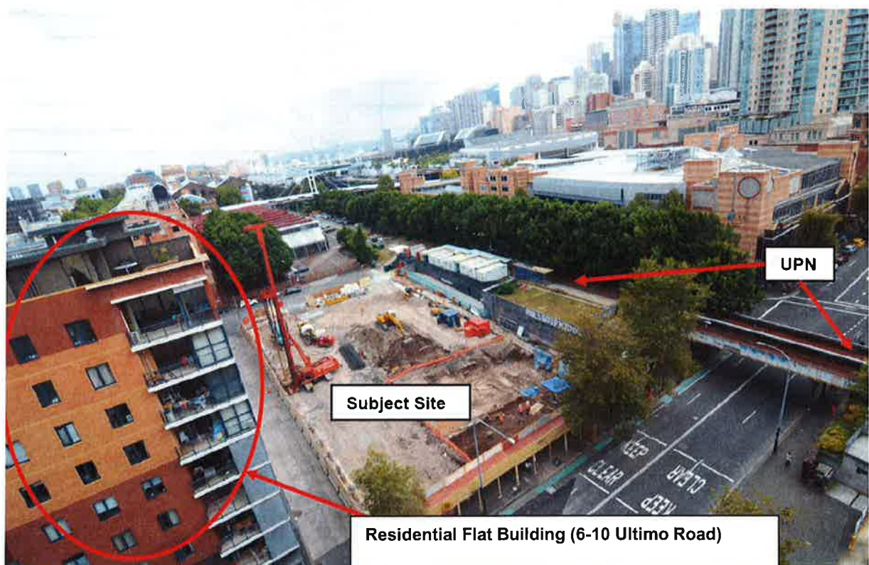
Figure 3: Subject Site Viewed from the Southern Side of Ultimo Road
