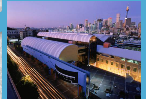
Powerhouse Museum Philip Cox Richardson Taylor and Partners/Lionel Glendenning
