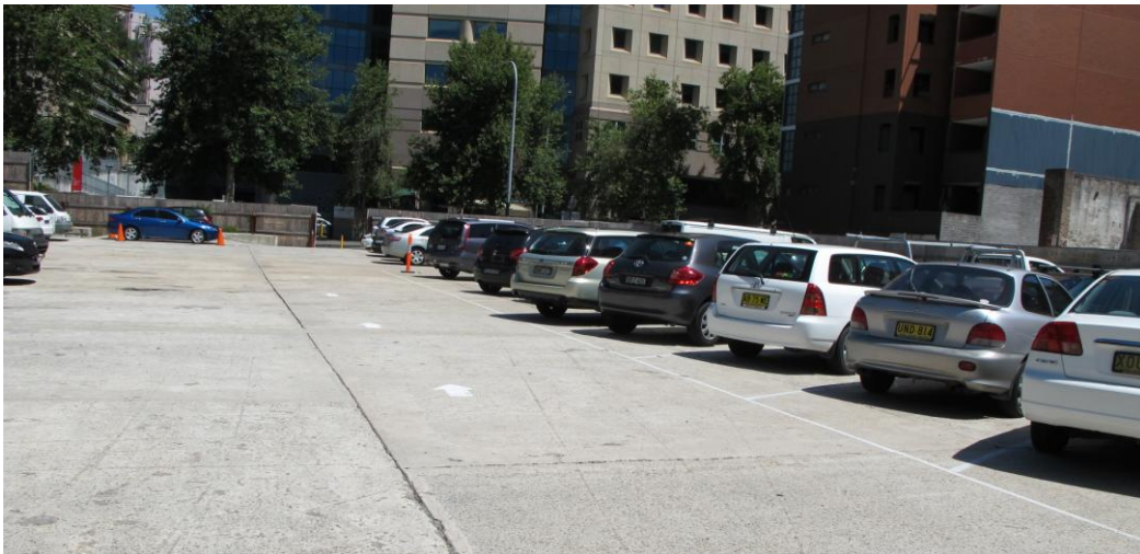
Figure 1.4: View looking south towards Ultimo Road inside the carpark. This surface of the carpark is a flat area raised above the current street level.
