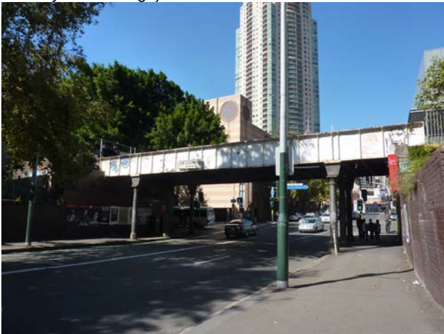
Photograph 2.3 The bridge over Ultimo Road (Ultimo Street Railway Underbridge).
