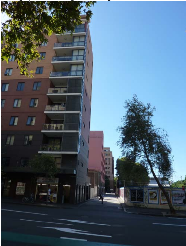
Photograph 2.7 Looking north along Omnibus Lane from Ultimo Road.
