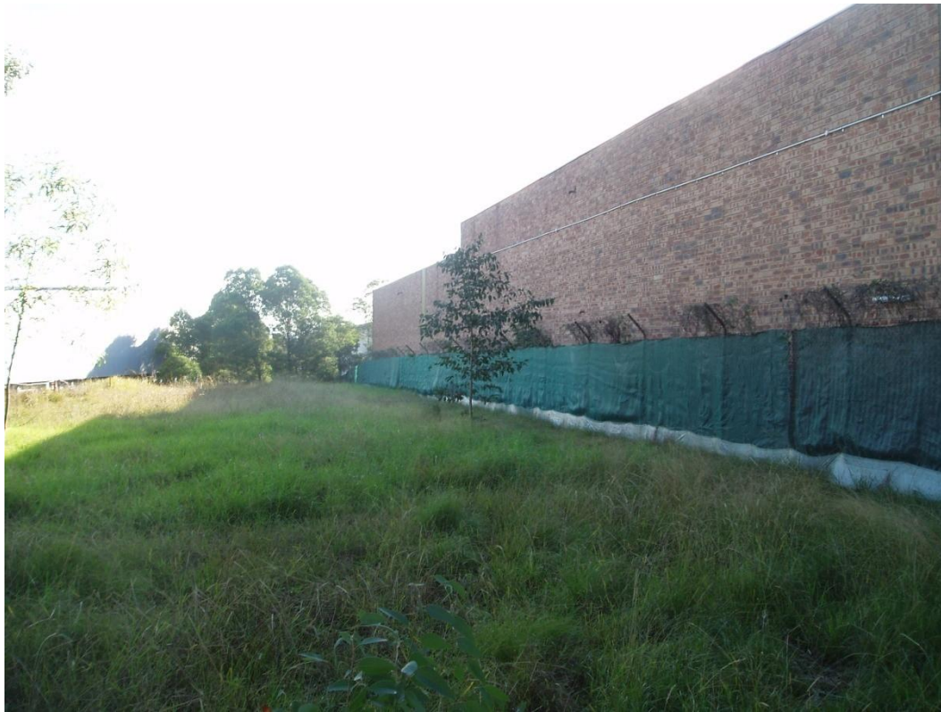
Photograph 11: Back Wall of Adjacent Property
