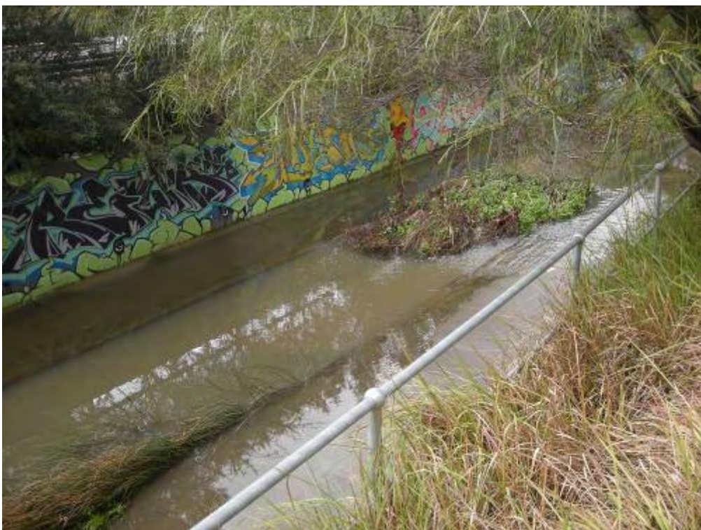
Plate P10: Byrnes Creek channel – section between Shaddock Avenue & Miller Road
