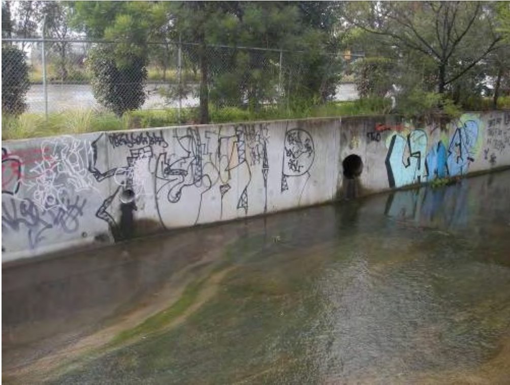
Plate P3: Byrnes Creek channel north side – east of Shaddock Avenue
