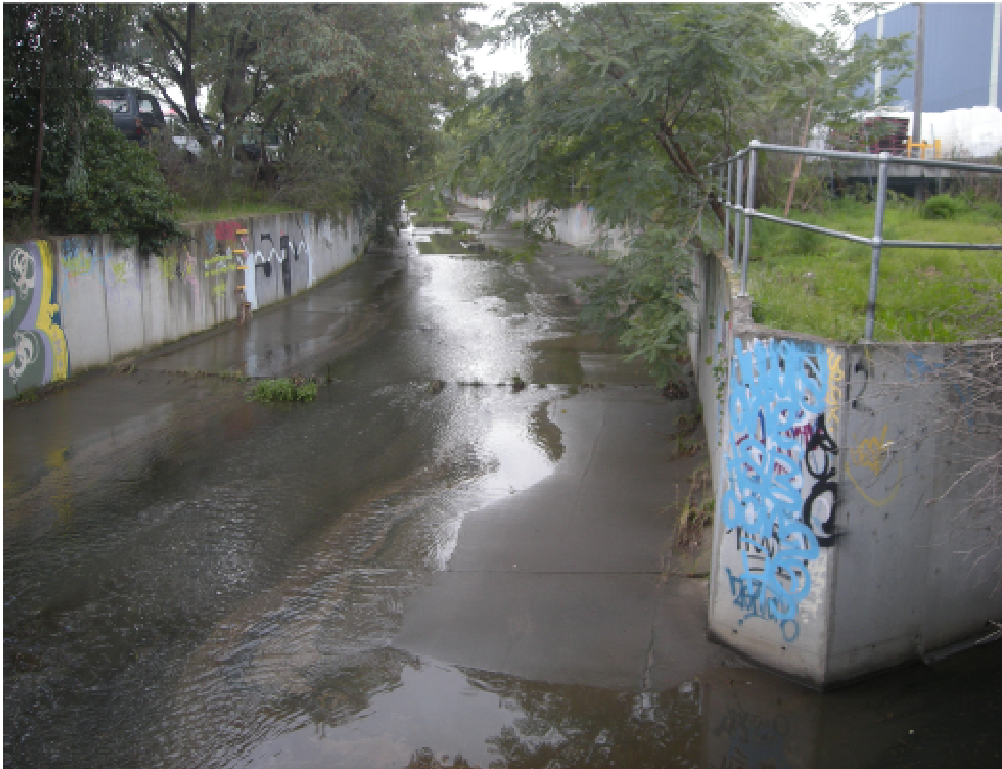
Plate P5: Byrnes Creek channel – junction with second channel looking upstream
