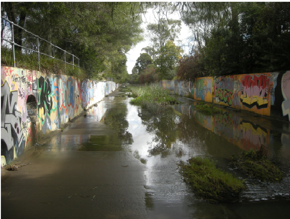
Plate P8: Byrnes Creek channel – section between Shaddock Avenue & Miller Road looking downstream
