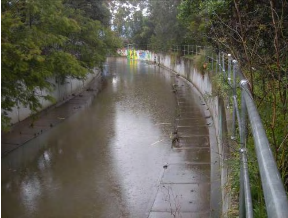
Plate P11: Byrnes Creek channel – view from north of Christina Road crossing looking downstream
