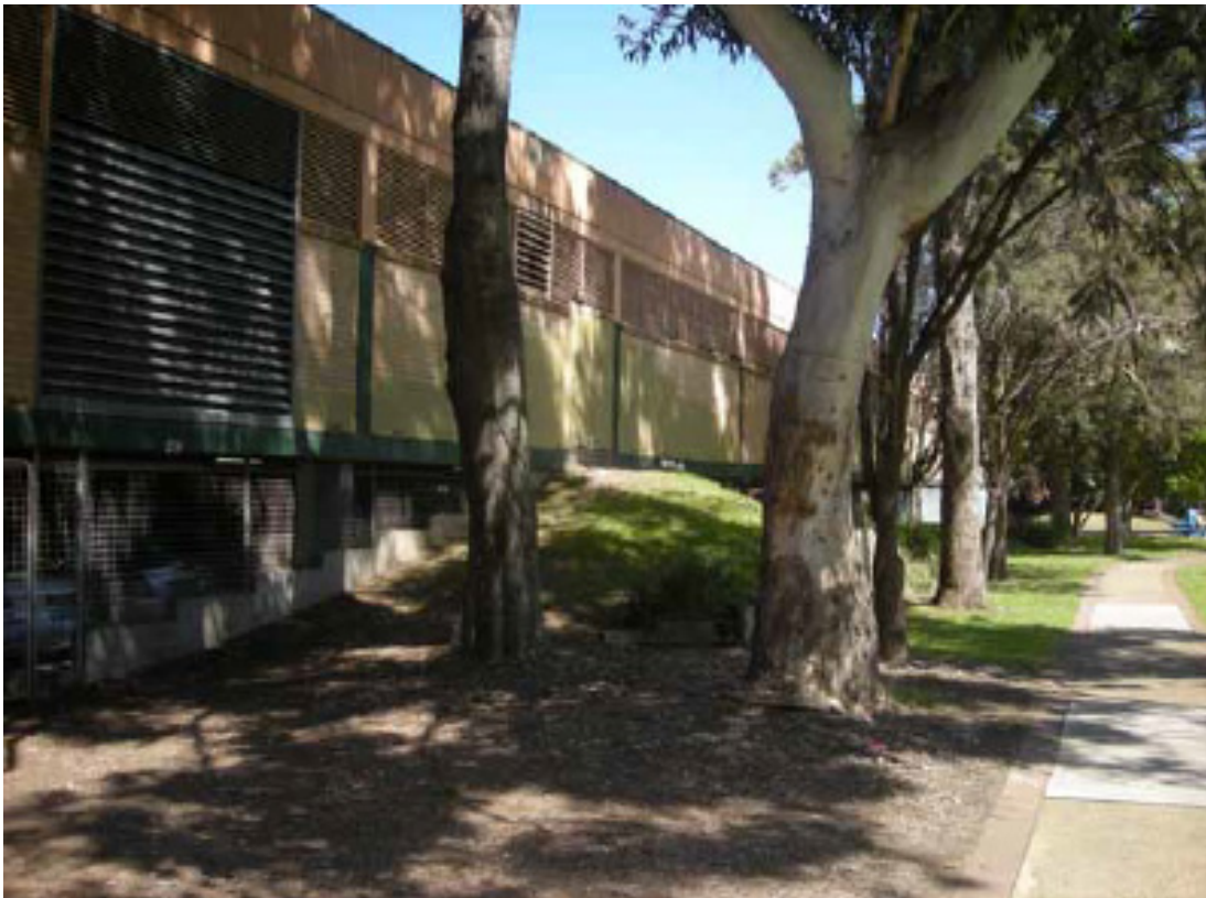
Figure 6 – Photograph showing the existing relationship of the centre to Eastlakes Reserve
