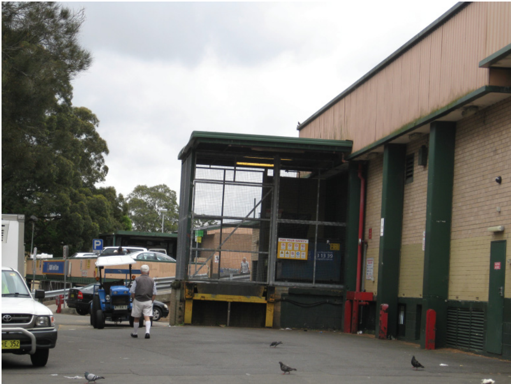
Photo 4 - Existing Woolworths loading dock facilities
