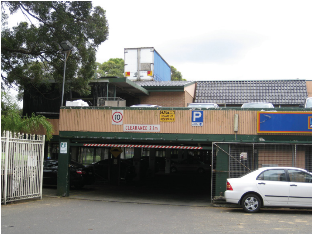
Photo 2 - Existing entry to basement car park from Barber Avenue
