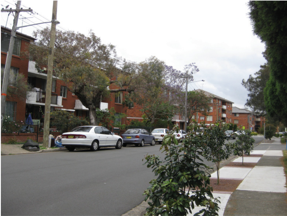
Photo 5 - View looking south along Barber Avenue
