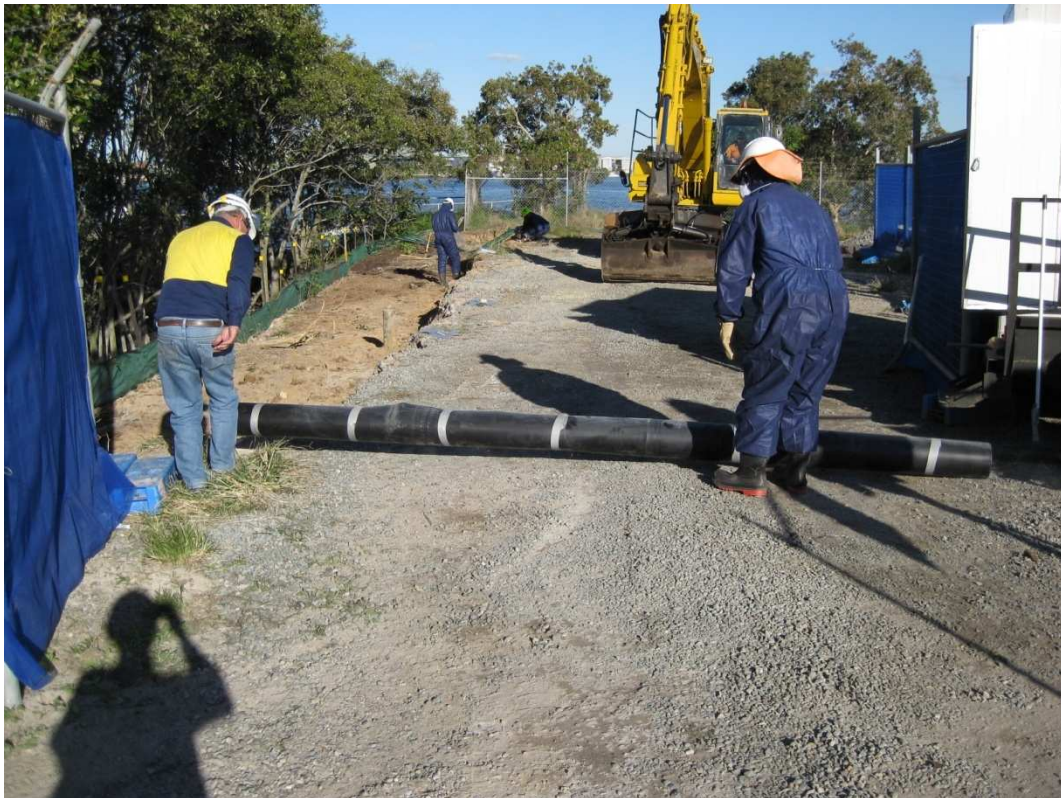
HDPE roll to be deployed
