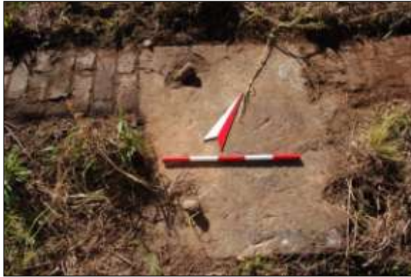
Figure 38: Brick annulus of Northern Gasholder, detail of concrete base for upright stanchion
