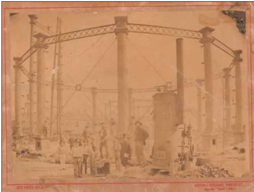
C. Lewis Construction Team Building Largest Gas Holder in Haymarket First Light: 150 Years of Gas
