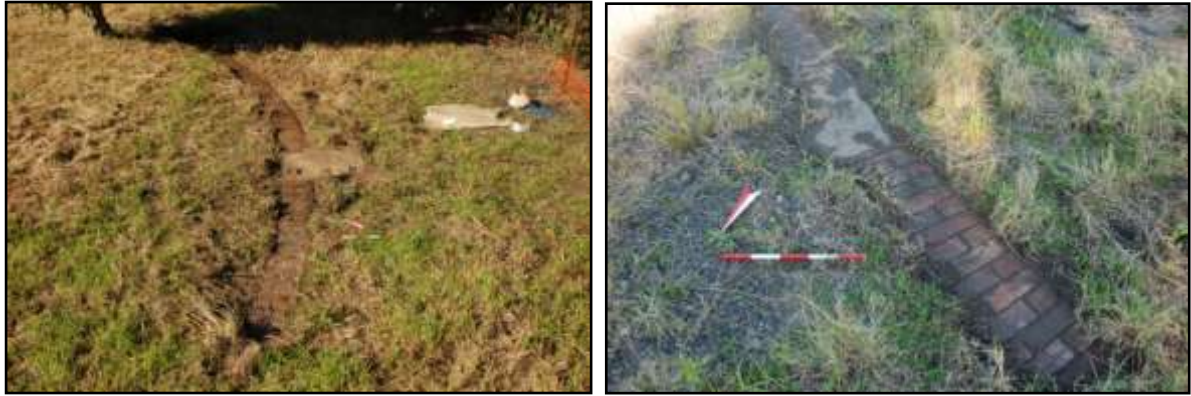
Figure 7: Remnant brick annulus from northern gas holder as seen during excavation works in June 2010. (photos by Gina Scheer and Franz Reidel)
