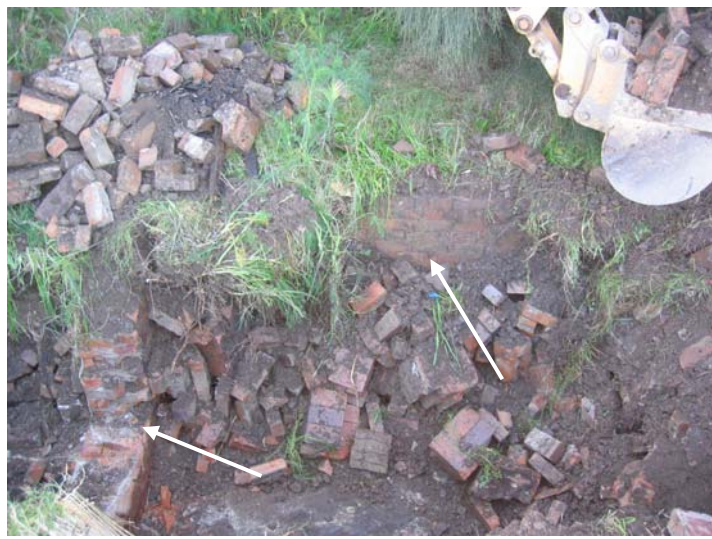
Photo 74 (Aug 06) – Retaining walls and fill in testpit TP12
