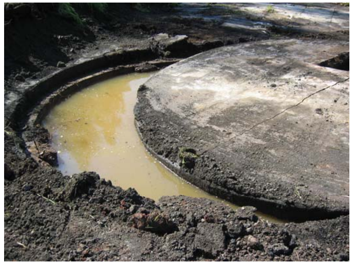
Photo 52 (Aug 06) – Water within the tar well (floating on top of tarry waste)
