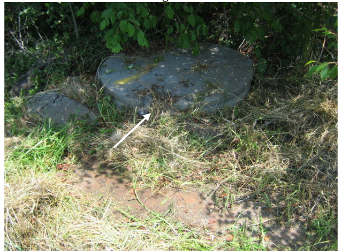
Photo 16 (Dec 06) – Cable pit servicing communications cables in north west site area
