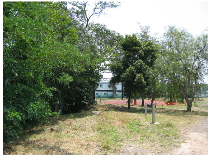
Photo 22 (Dec 06) – Trees located along top of embankment, in south western site area
