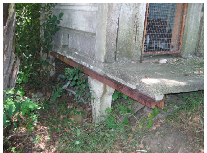
Photo 18 (Dec 06) – Old electrical shed on embankment, south of the existing gasholder
