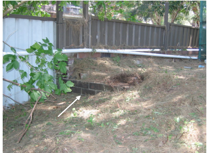
Photo 14 (Dec 06) – Additional level of brickwork on top of retaining wall area
