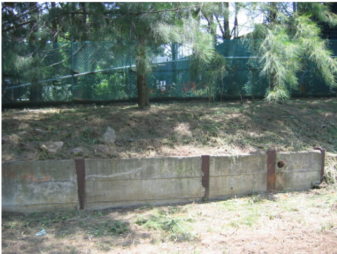
Photo 15 (Dec 06) – Note difference in levels in north west area. Site is level with Burren Street, however area on top of retaining wall (and Stabling Yard surface level) is ~1.5m higher
