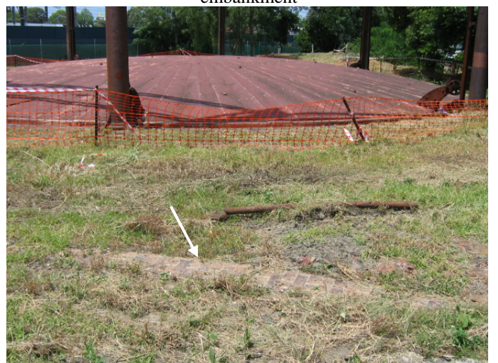
Photo 6 (Dec 06) – Annulus of demolished gasholder remains in situ, to the north of the existing gasholder
