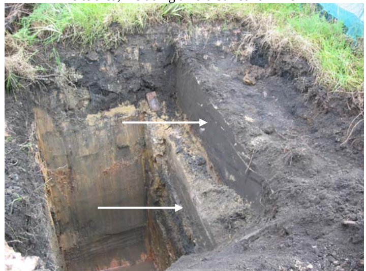
Photo 72 (Aug 06) – Fill profile in testpit TP10, on northern site boundary, including two stepped retaining wall
