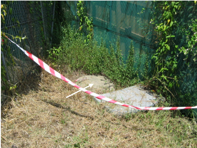
Photo 19 (Dec 06) – Sydney Water sewer pit located in south west corner of site
