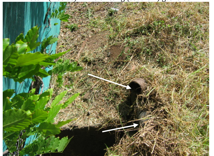
Photo 4 (Dec 06) – Sydney Water sewer line located under embankment (1m from fence which adjoins Burren St properties). Disused gasworks pipework also buried in embankment
