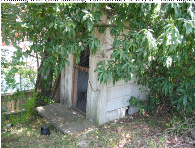
Photo 17 (Dec 06) – Old electrical shed on embankment, south of the existing gasholder
