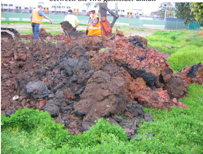
Photo 41 (Aug 06) – Material excavated from area adjacent to northern gasholder annulus
