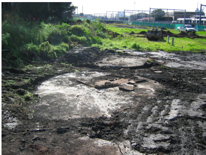
Photo 49 (Aug 06) – Two tar pits with concrete lids, in north west site area
