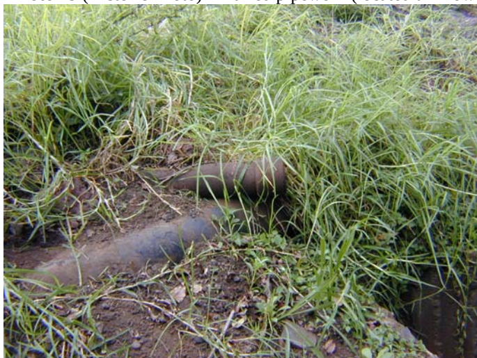
Photo 81 (Historic Photo) – Buried pipework (located unknown)
