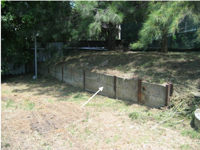
Photo 13 (Dec 06) – Concrete retaining wall (with steel rails)
