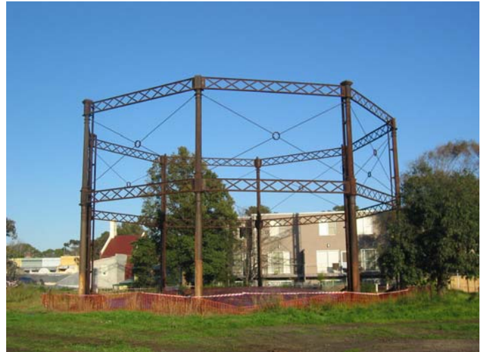
Photo 2 (Dec 06) – The existing (southern) gasholder
