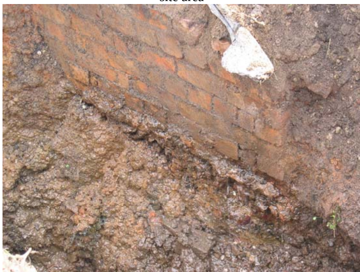
Photo 77 (Aug 06) – Brickwork and tars beneath the former retort house in testpit TP15
