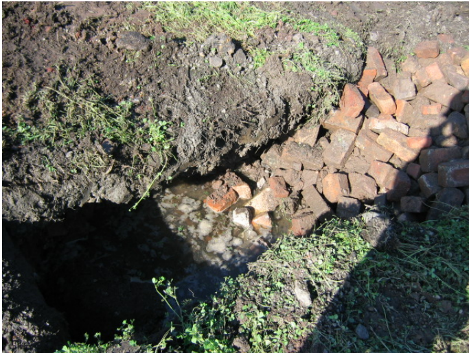
Photo 37 (Aug 06) – Demolition materials and significant perched water within northern gasholder annulus (MG04)
