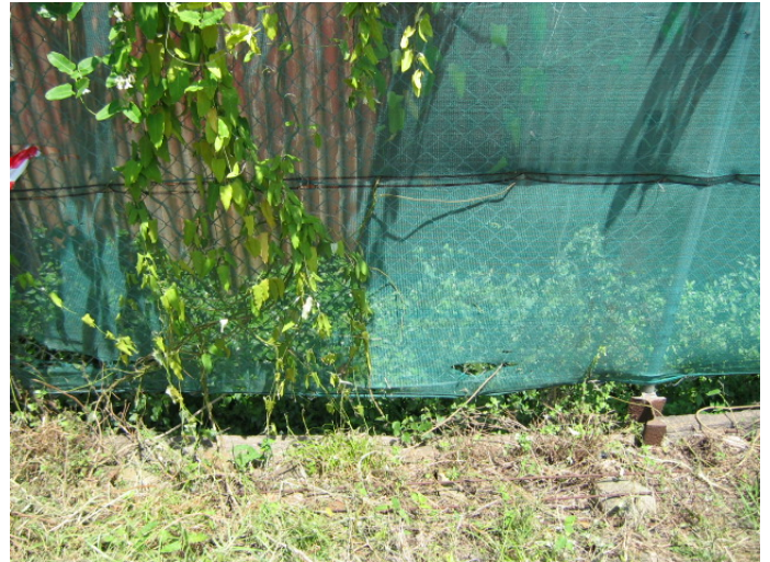
Photo 20 (Dec 06) – Open drain located between western fenceline, and rear of Burren St properties. Drain is in poor condition and overgrown, and lies approx 1m below embankment level
