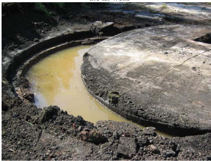
Photo 52 (Aug 06) – Water within the tar well (floating on top of tarry waste)
