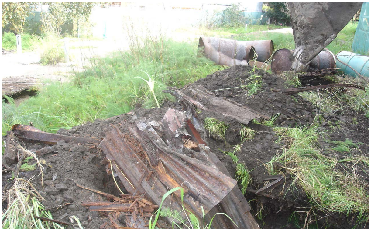
Photo 20 Subsurface conditions of Retaining Wall Area at sample location TP18. Indicative material of Gravel, Sand and Demolition Wastes.
