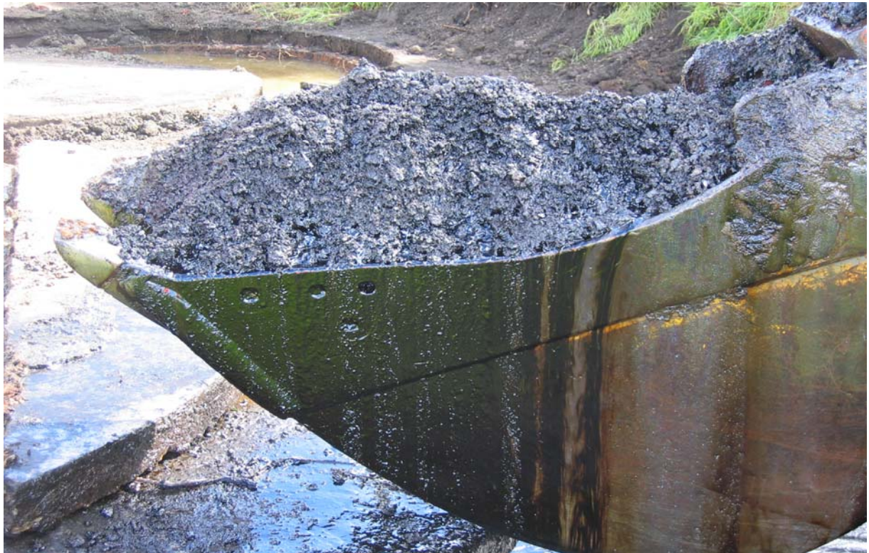
Photo 13 Tar Well #2 showing coal tar and gravel contents.
