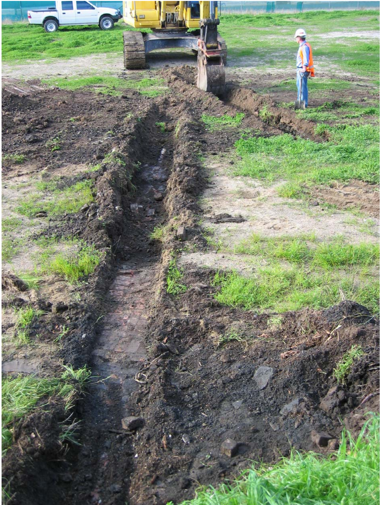
Photo 16 Facing south toward former Retort House area showing historic brickwork. Shows sample location MG09A (foreground) and MG09B (background with excavator).
