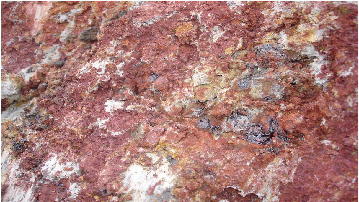
Photo 23 Subsurface conditions showing free tar in deep red/grey natural clays at sample location MG08 at 3.1mbgl.
