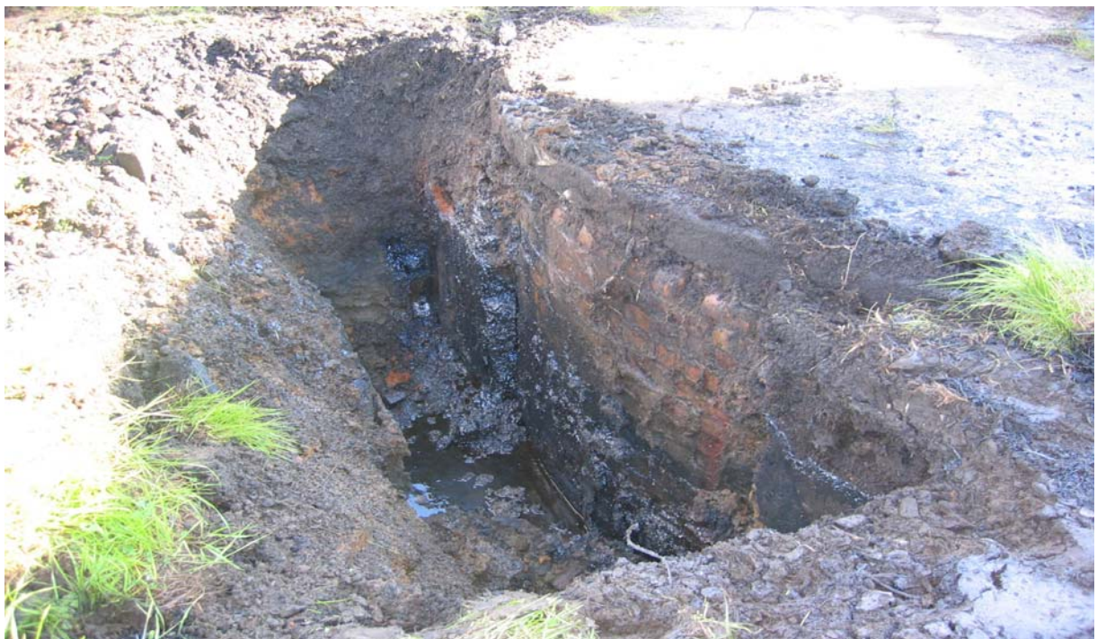
Photo 14 Facing west toward sample location MG06 at Tar Well #2 showing tar seepage from brickwork.
