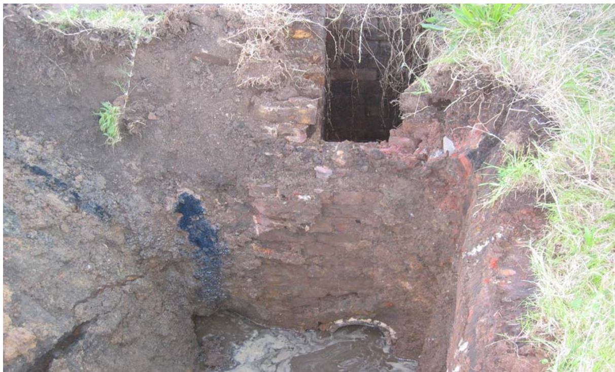
Photo 15 Facing west toward sample location RP and brick Retention Pit.
