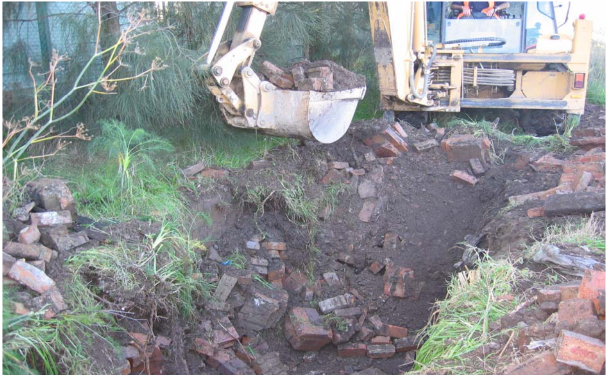
Photo 21 Subsurface conditions of Retaining Wall Area at sample location TP12. Indicative material of Gravel, Sand and Demolition Wastes.
