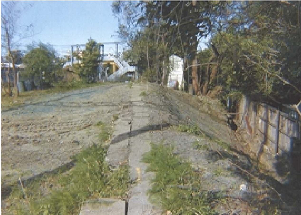
Plate 1: Elevation difference between the Former Gasworks Area and the adjacent residential properties. The open concrete drain is also visible.
