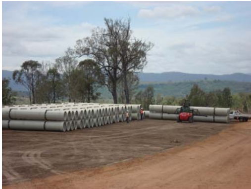
Plate 1. Pipe laydown yard.
