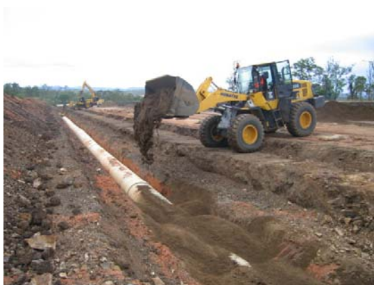
Plate 8. Backfilling.
