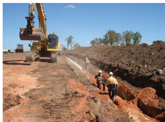
Plate 9. Compacting.
