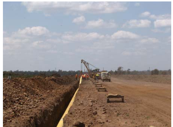
Plate 7. Pipe laying.
