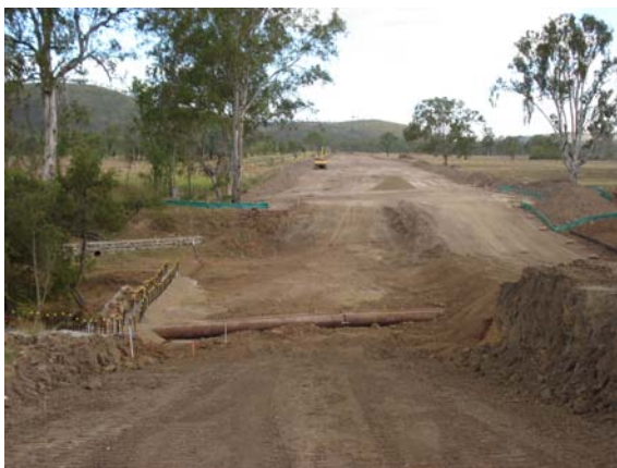
Plate 5. ESC – sediment weir and silt fence.
