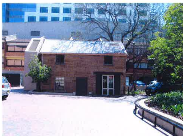
Figure 3.19 Perth House Stables, East Elevation [Source: CM+, October 2004]
