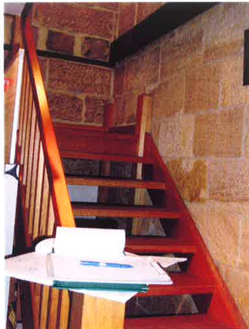
Figure 3.23 Perth House Stables, recent stair addition. [Source; CM+, October 2004]
