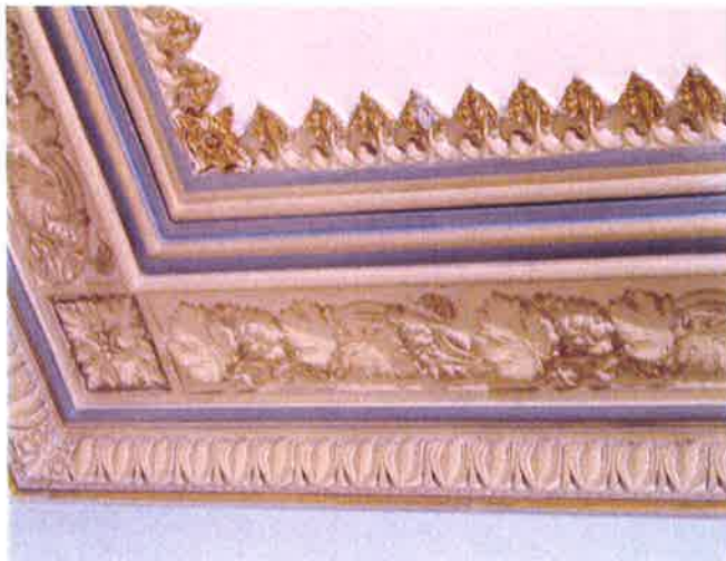
Figure 3.15 Perth House, Room 7 showing decorative plaster cornice detail. [source; CM+, October 2004]
