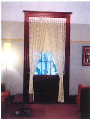
Figure 3.8 Perth House, Room 3 window showing cedar joinery [Source: CM+, October 2004]
