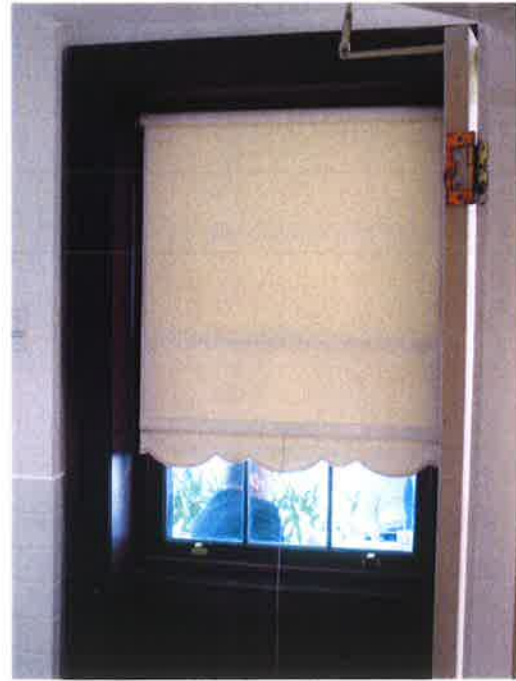
Figure 3.14 Perth House, window in Room 6 – now toilet facility. Windows are smaller in scale than those in the front rooms. [Source: CM+, October 2004]
