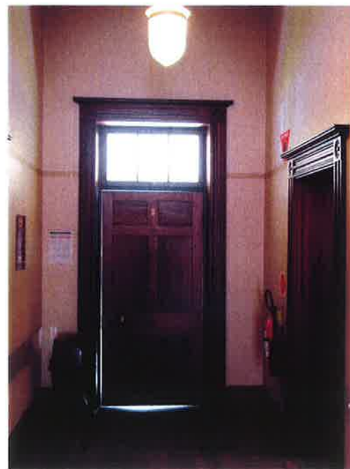
Figure 3.6 Perth House, Hall interior showing six panel cedar front door and fanlight [Source: CM+, October 2004]
