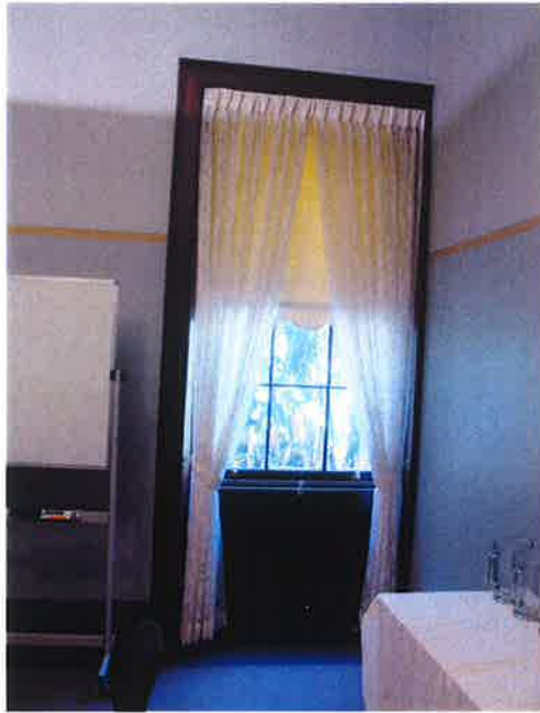
Figure 3.11 Architraves in Room 4 have a simpler profile to those in the front rooms. The wall is a later addition [Source: CM+, October 2004]
