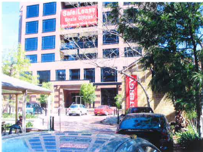
Figure 3.26 Office Tower, south of Perth House [Source: CM+, October 2004]
