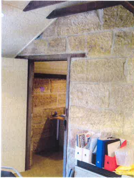
Figure 3.24 Perth House stables, Upper floor, showing two rooms in former loft [Source: CM+, October 2004]
