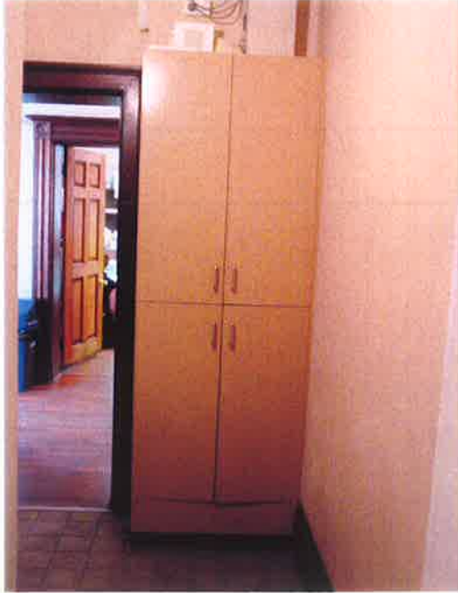
Figure 3.13 Perth House, distribution cupboard located in Room 6. Room converted to accommodate toilet facilities [Source: CM+, October 2004]
