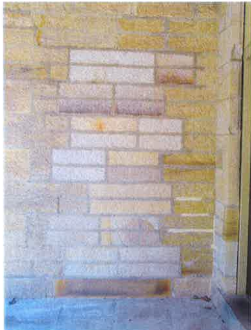
Figure 3.18 Perth House, Verandah room (R6) with later door opening infilled [source CM+, October 2004]
