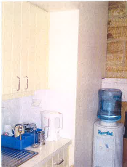
Figure 3.22 Perth House Stables, Ground Floor, recent kitchenette addition in the former animal stall. [Source; CM+, October 2004]
