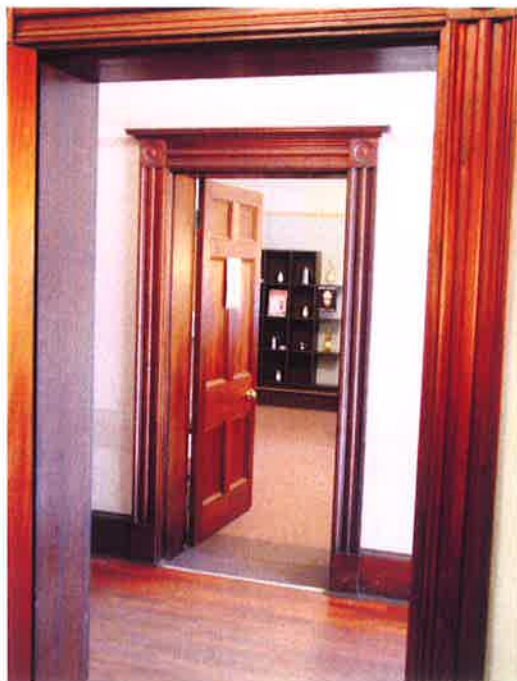
Figure 3.5 Interior of Perth House, showing cedar joinery and door architraves [Source: CM+, October 2004]
