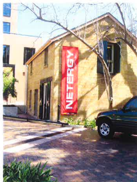
Figure 3.20 Perth House Stables showing North and East Elevations [Source: CM+, October 2004]
