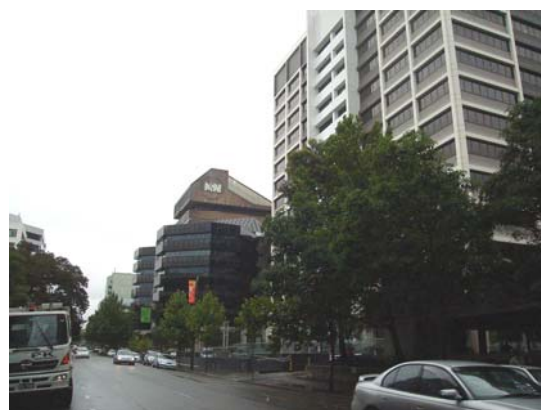
Photo 2 North side of George Street looking west
