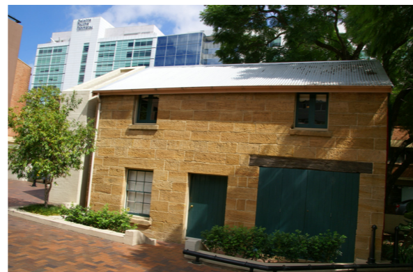
Existing building to west of forecourt
