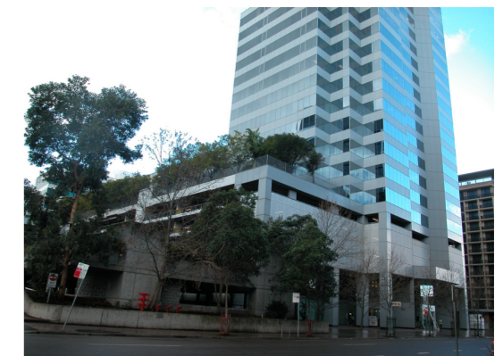
3. 150 George Street viewed from George Street
