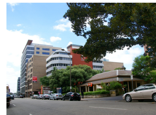
7. View of Perth House, 91, 93 & 95 George St viewed from George St looking East
