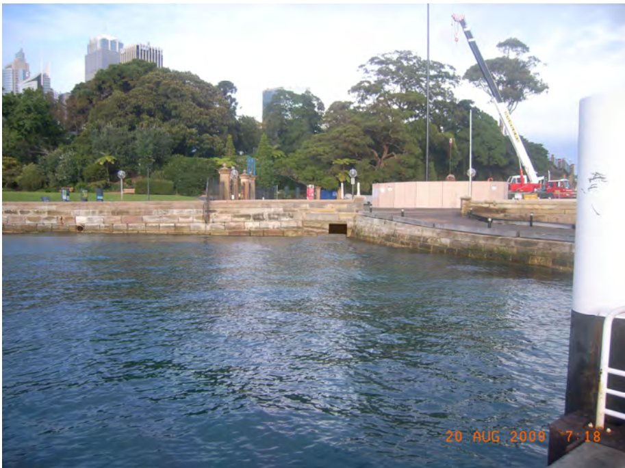
Figure 7-4 View of proposed outlet from Man O' War Jetty at high tide
