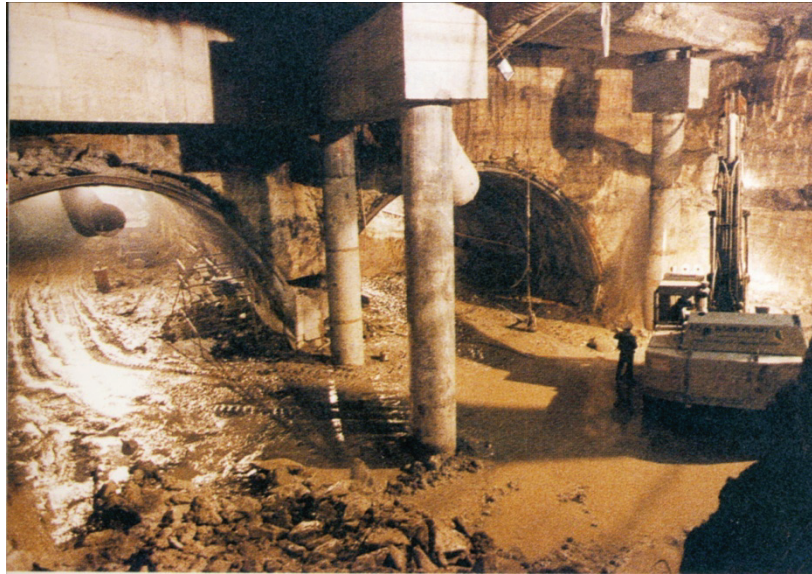
Looking south beneath the forecourt, with the northern ends of the two southern land tunnels and the new columns and beams clearly shown.
