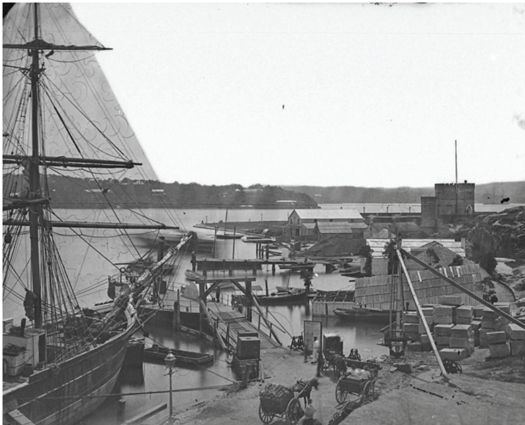
Figure 4: Western side of Fort Macquarie showing sandstone blocks being quarried from the Tarpeian Cliff ~1870
