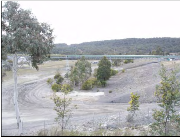
Figure 7.1 View of study area A looking north
