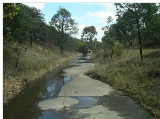
Area 2 Drain (concrete channel) with planted vegetation on embankments
