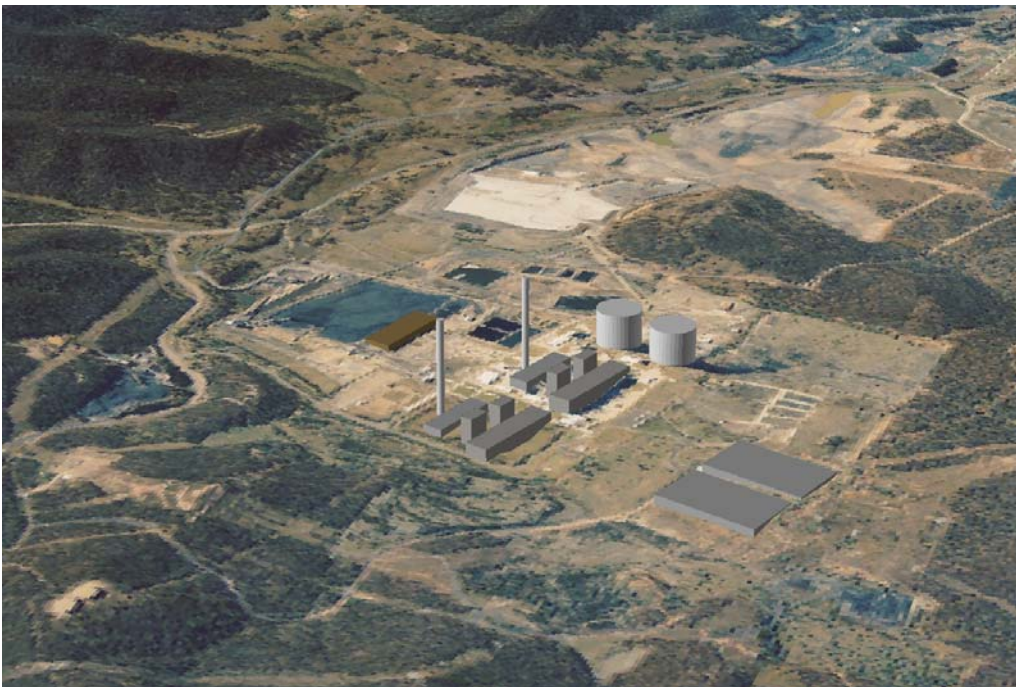
■ Figure 11-7 View of Power Station Extension (USC coal) to the north east
