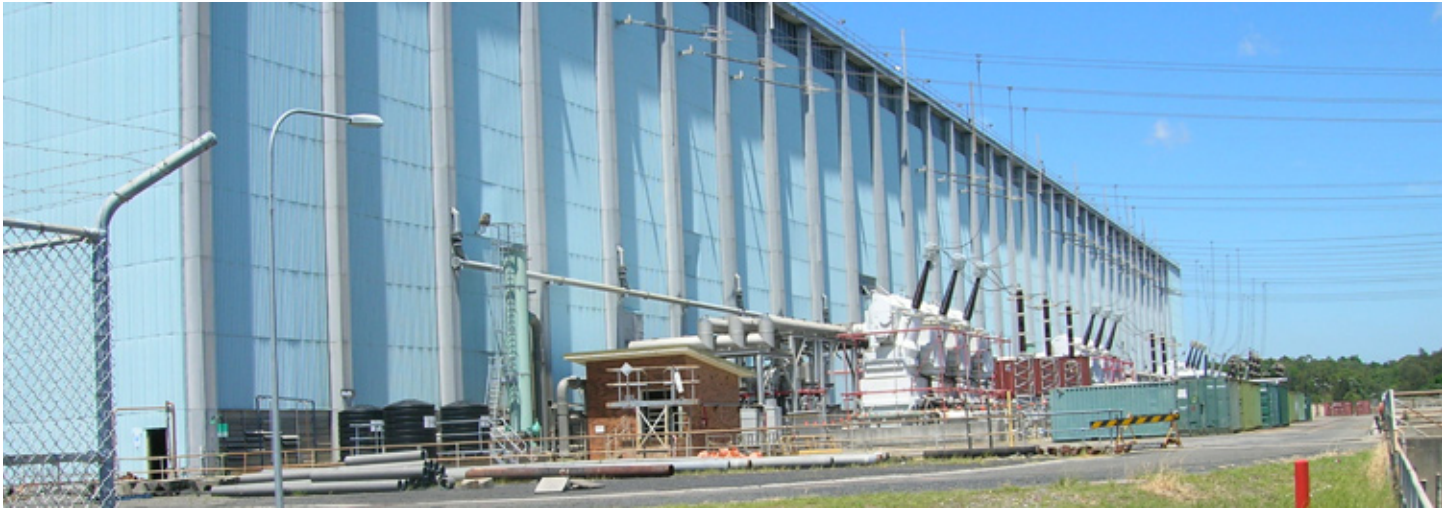
External view of Turbine Hall
