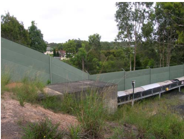
Plate 3.3 – Section of the MV conveyor passing through a culvert
