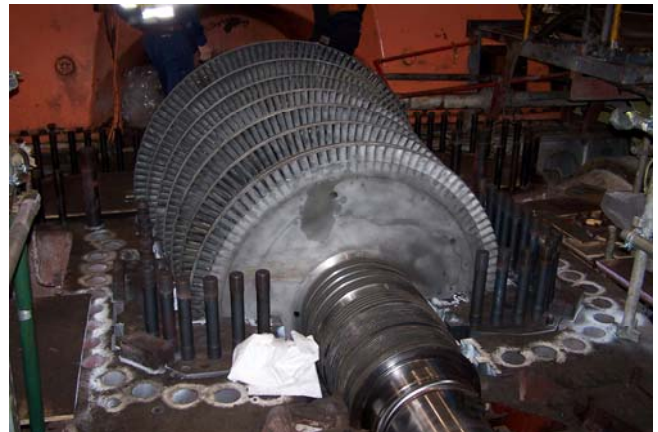
Plate 3.1 – IP turbine blades
