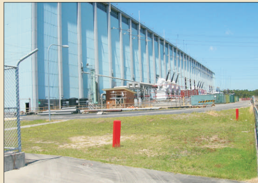
External view of turbine hall
