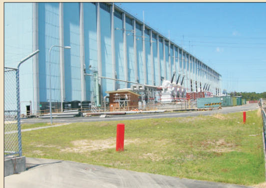
External view of turbine hall
