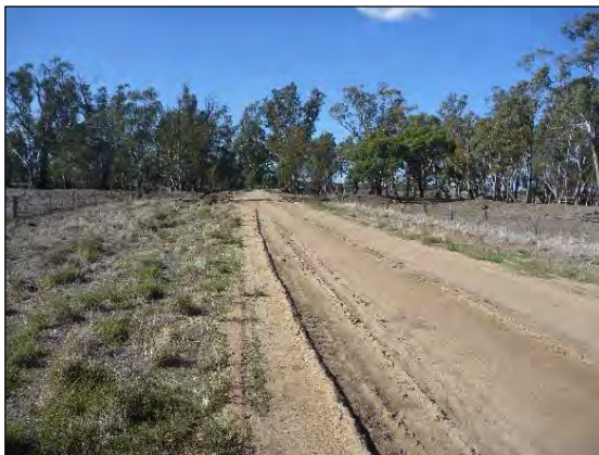
Figure 5.1 Recently graded road facing north
