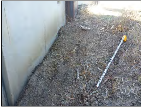
Figure 5.7 Shell scatter next to concrete support
