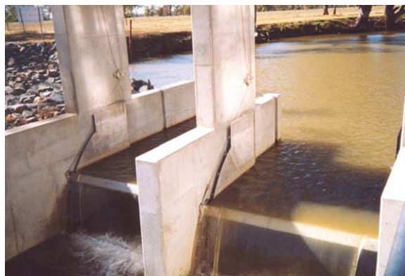
Figure iv: Photo of typical Aluminium Tilting Gate Regulator
